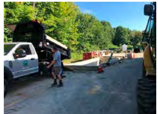
DPW site work for scale at Transfer Station
