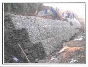
What is a gabion basket or gabion retaining wall? Gabions and vegetated gabions
